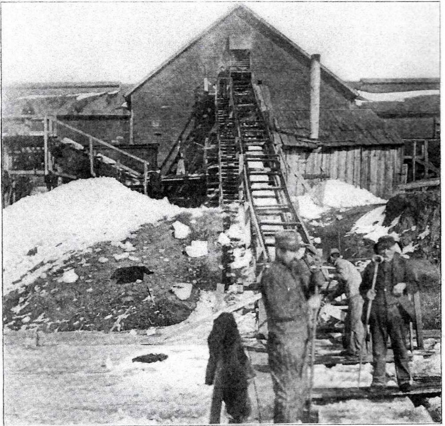
FIG. 29. UNDERSHOT ELEVATOR AND CAR LOADER. HASTINGS ICE COMPANY, HASTINGS, NEB.
